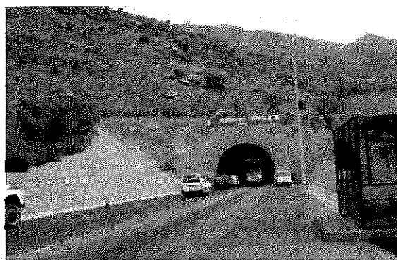
Kohat Tunnel North Portal
